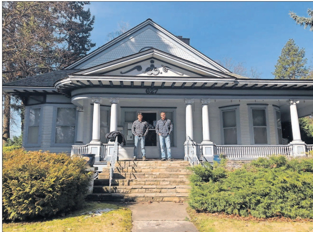
John Swallow, left and Rob Johnston will be helping with the renovation construction for the future Music Conservatory of Coeur d'Alene, former Romer house.
